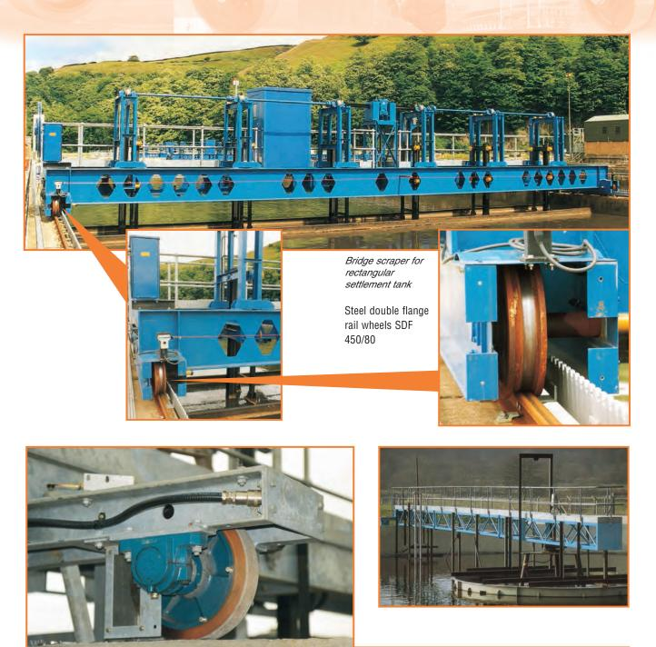
Half Bridge scraper for rotary settlement tank
