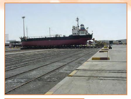
A ship lift and transfer dock system for removing ships from the sea and then transferring ships around the dock for repair and maintenance to take place. Three sizes of wheels are used througout the dock.
